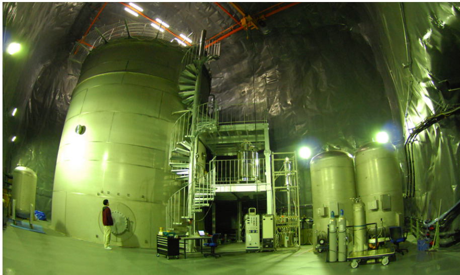
XMASS infrastructure in construction in the Kamioka mine
