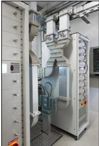
RF amplifier for FZD 10kW @1.3 GHz
