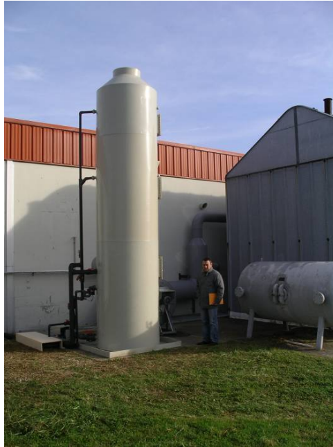
Figure 12: Gas scrubber outside the laboratory.
