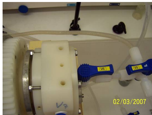
Figure 24: Distinct sulphur deposition on the pipe at the outlet of the cavity.
