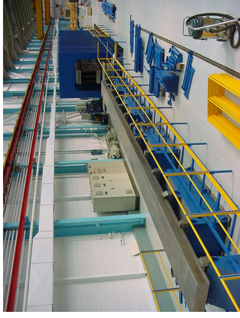
Shell-welding press for twin-aperture, 15-m-long LHC arc dipole magnets at Alstom/MSA
