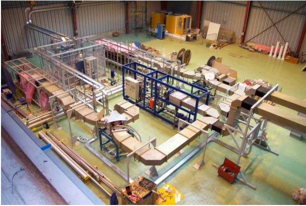
Figure 5 : View of the RF power system assembly
