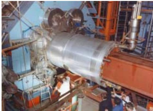
Fig 2. The Cello solenoid being inserted in the argon calorimeter and the iron yoke
