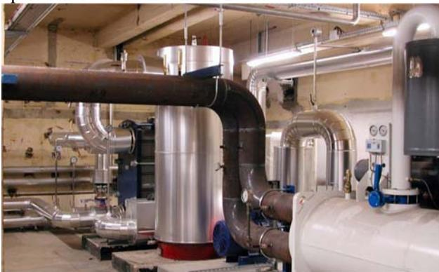
Figure 7 : View of the chilled water plant connected to the RFQ temperature control system.
