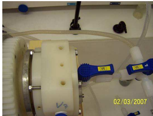
Figure 24: Distinct sulphur deposition on the pipe at the outlet of the cavity.
