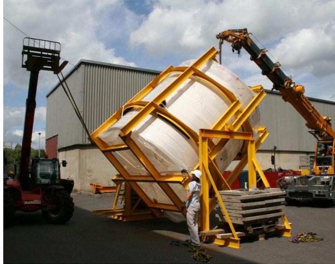
Figure 10.2: Gamma Catcher rotation, prior to enter in the tunnel leading to the laboratory. Special tooling was designed by Saclay. Two cranes were necessary to realize the operation safely.
