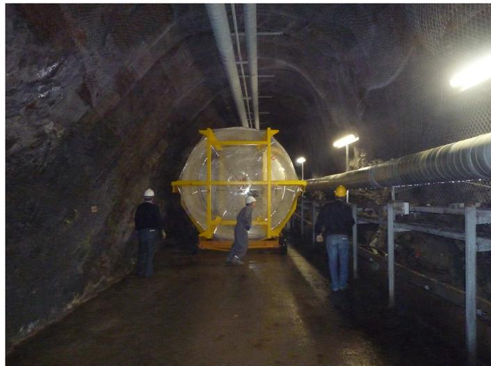
Figure 10.3: Gamma Catcher going down the tunnel. A crane secured the vessel from behind. The tunnel dimensions were very tight; we even had to break some rocks in order to let the Gamma Catcher go through. Two fake runs were performed before the real one.
