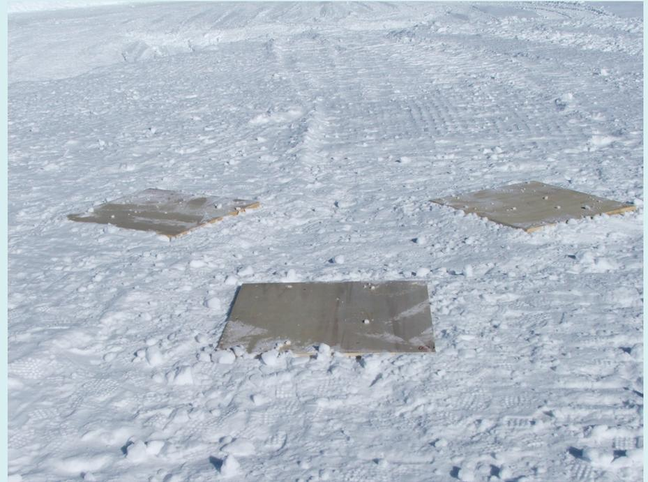
Wood base on the platform to prevent from sinking into the ice
