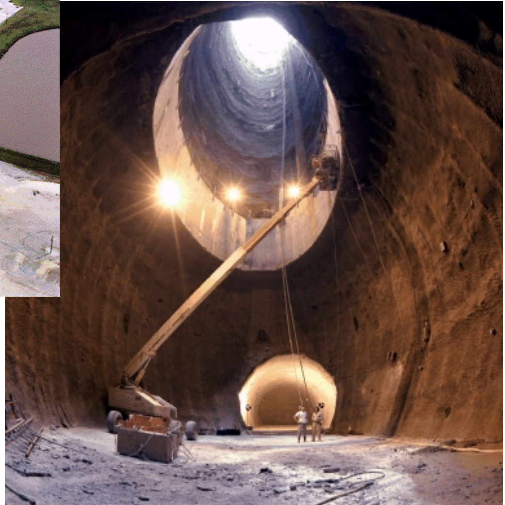
Bottom View of Main Shaft to SSC Tunnel
