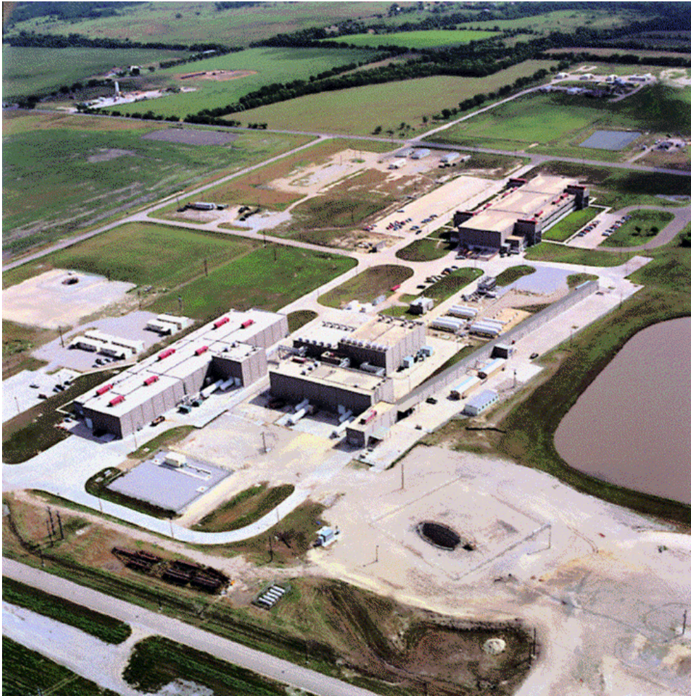
Aerial View of N-15 Construction Site Near Waxahatchie, TX
