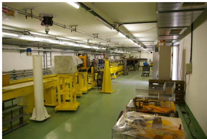
Figure 1. : CALIFES construction in CLEX building (December 2007).
