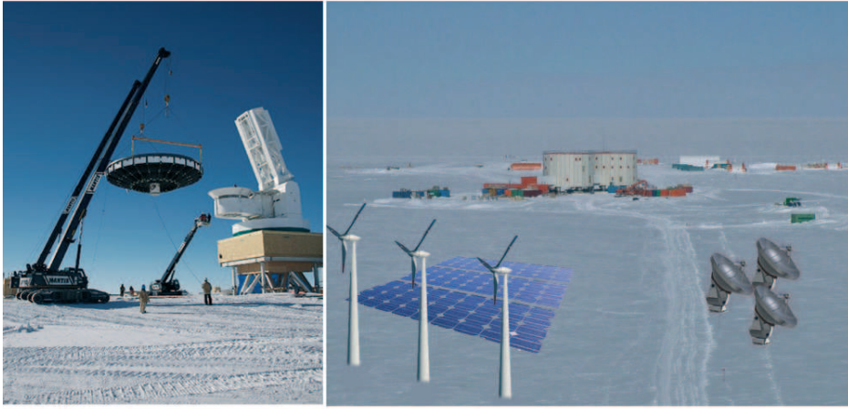
Fig. 11. Left: Deployment of the SPT at South Pole and required level of logistics. Right: View of a possible 3 \times 12 -m antenna interferometer at Dome C with renewable energy supply. The deployment of such telescopes at Dome C would require an important and costly upgrade of the current Concordia station.
