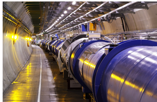
(b) View of the hadron accelerator (blue modules) inside the underground tunnel.
