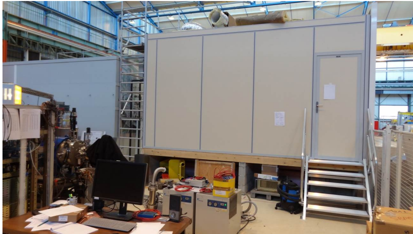
Figure 13.7: The laser hut built in the GBAR zone (the positron trap can be seen on the left); picture taken during the installation of the air conditioning unit.
