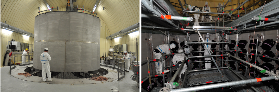
Figure 6.4: Left: Buffer vessel integration. Right: Installation of the Inner Detector PMTs.
