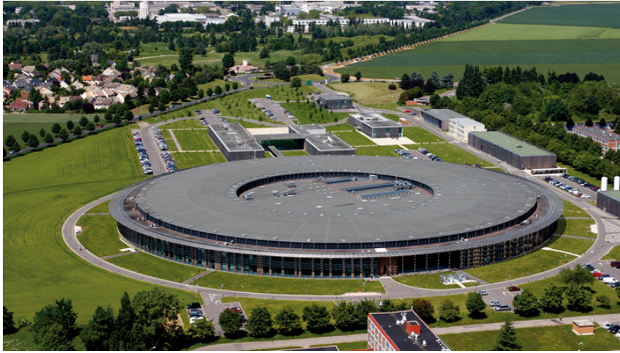
Figure 5.1: The Soleil Synchrotron Facility. The electron's accelerator is located inside the circular building.
