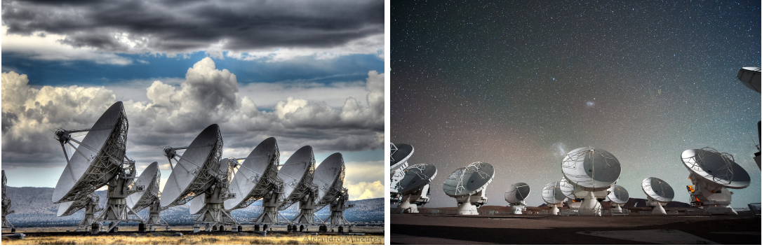
(a) The Very Large Array radio telescope is an array of 27 antennas of 25 m each. (b) The ALMA radio telescope. Placed at more than 5000 m height in the Chilean desert of Atacama, it is constituted by 66 antennas of a diameter varying from 7 m to 12 m.
