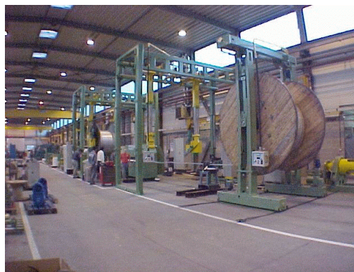
Fig. 2. Construction of the Continuous Electron Beam Welding Plant for the CMS conductor reinforcement.
