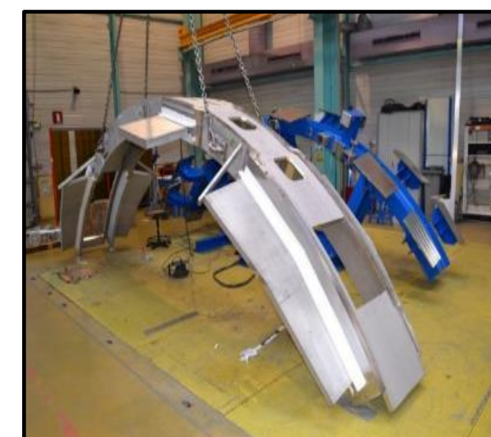
Structure inter-bobines JT-60SA
