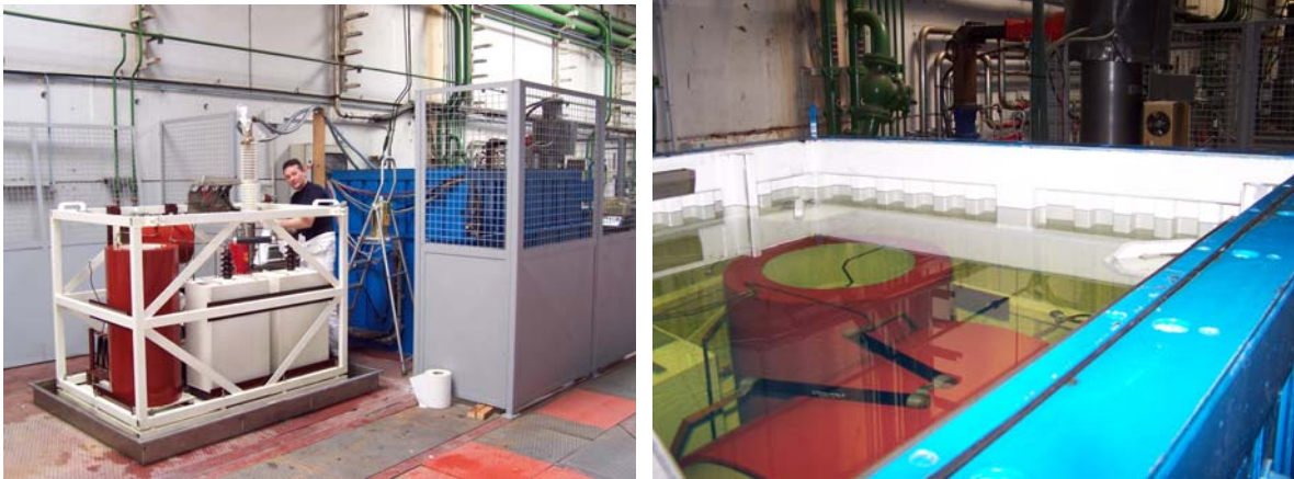
Figure 4: After repair and cleaning, modulator components are transferred in the oil-tank refilled with 4300 litres of new oil.
