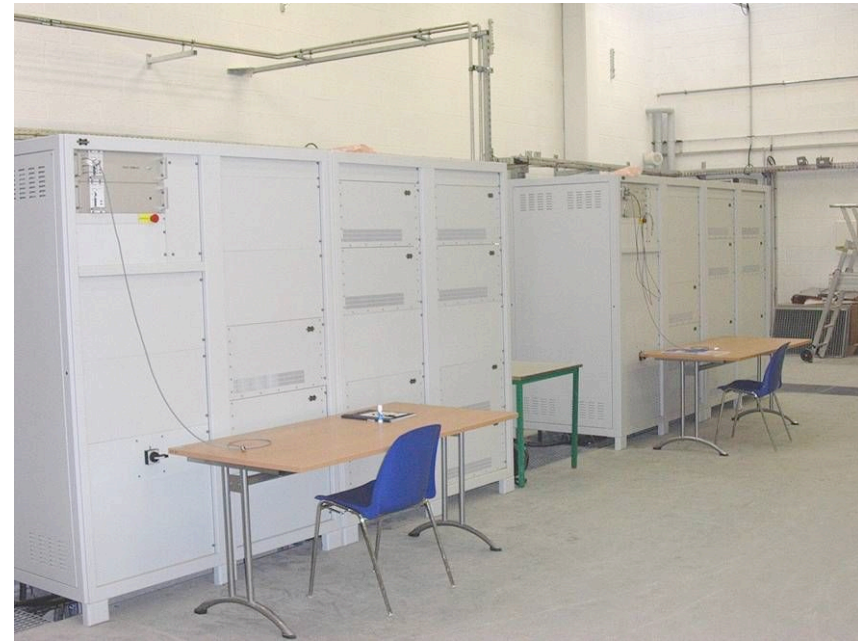
Dipole power supplies (Bruker, 3Hz) (2 x 560 A / 1000 V)
