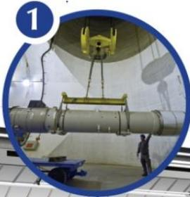
**39 dipole magnets replaced**
