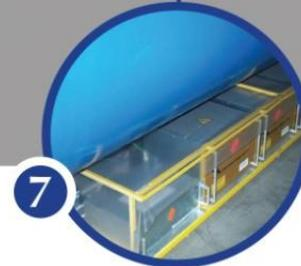
**New longitudinal restraining system for 50 quadrupoles**
