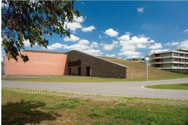
The facility building
