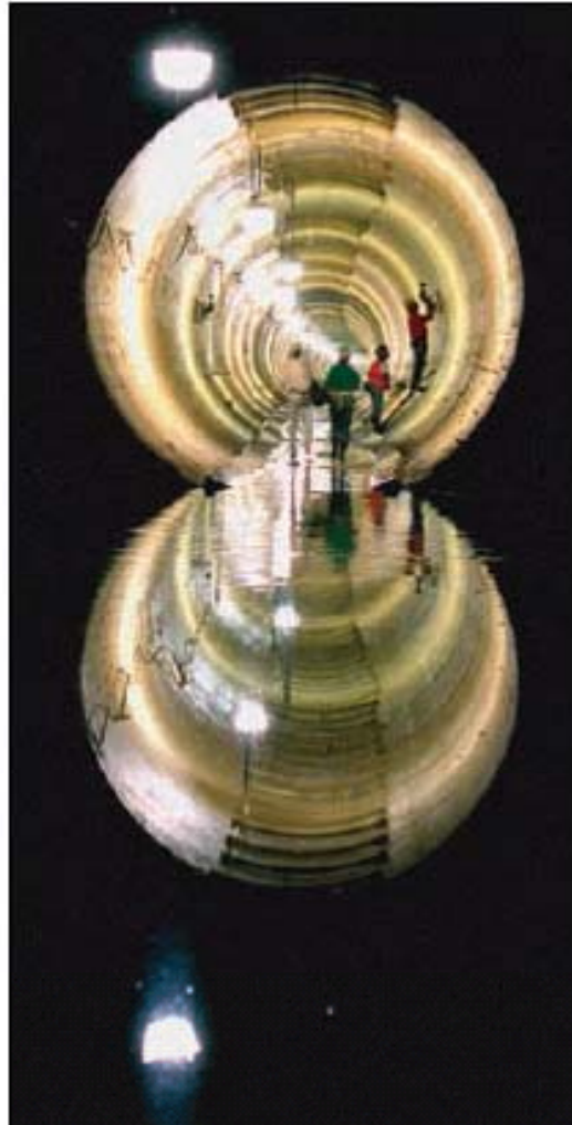
Terminated Texas tunnel. The SSC was abandoned after about 25% of the tunnel for the 87-kilometer-circumference large collider ring had been bored.
