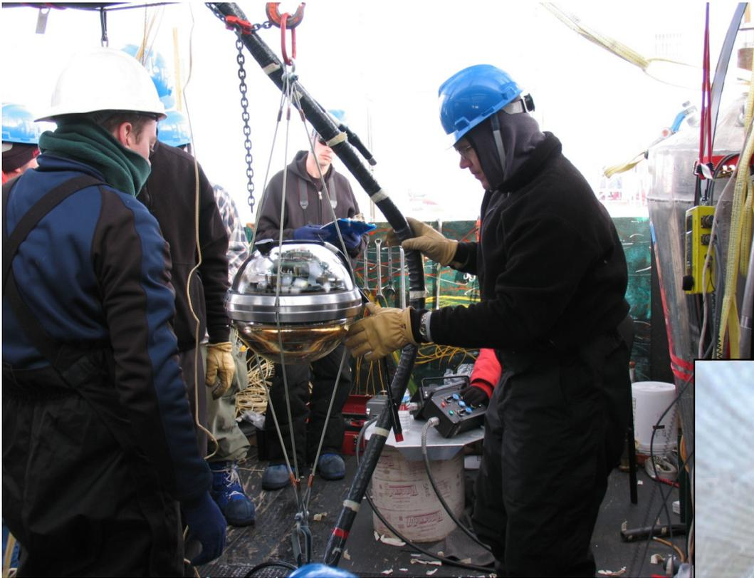
60 Digital Optical Modules on a string installed in 20 h
