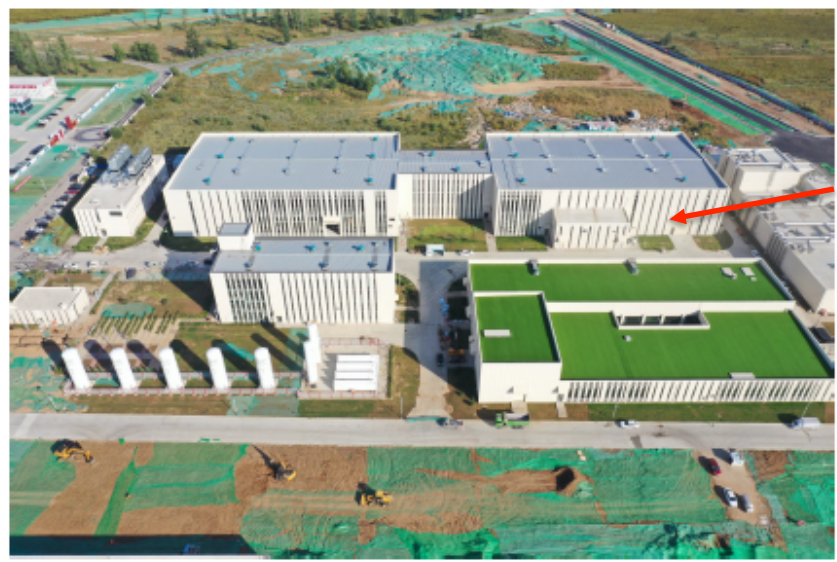
Bird view of IHEP New SC Lab under construction: 4500 m2
