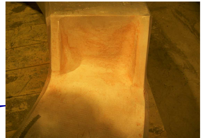
detections 3a and 3b (repaired)
